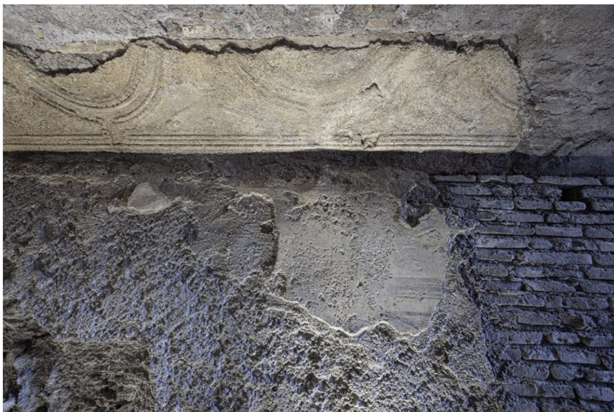
Remnants of the stucco on the originally marble-clad on the passageway's walls. Photo credit: Simona Murrone/Colosseum Archeological Park
